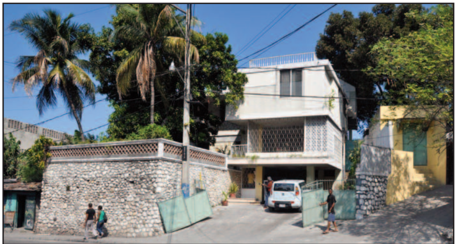
Before the Earthquake (house of the author's uncle)
